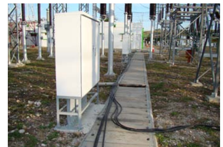
Simple fiber optic cable installation
