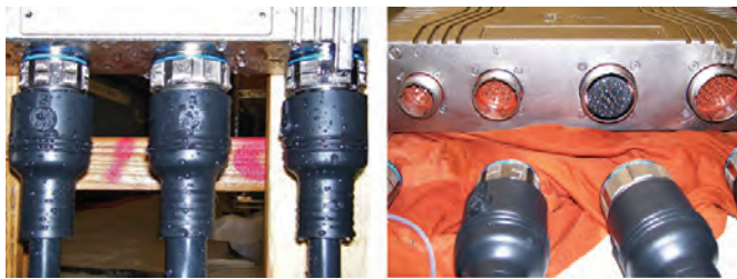
Figure 12. Water ingress testing for IP6x: pre-inspection (left) and post-inspection (right)
