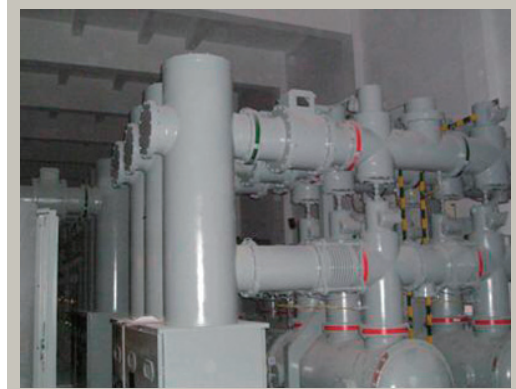
Figure 2. PCS-9250 series ECT/EVT for GIS application
