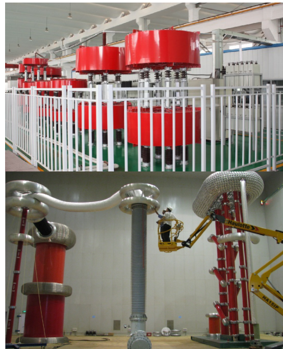
Figure 16 large current and high voltage test lab
