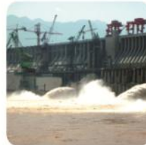
Largest Hydro Generation Three-Gorge Dam Power Plant
