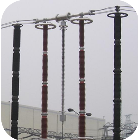
2*360 MVA SVCs & 2*390 MVA CSRs in 750kV Substation
