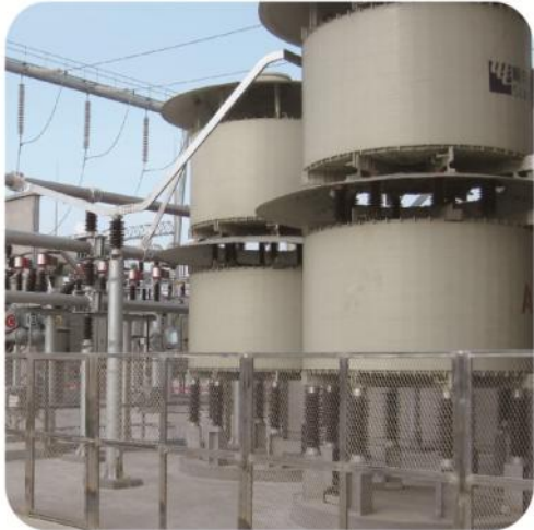
2*360 MVA SVCs & 2*390 MVA CSRs in 750kV Substation
