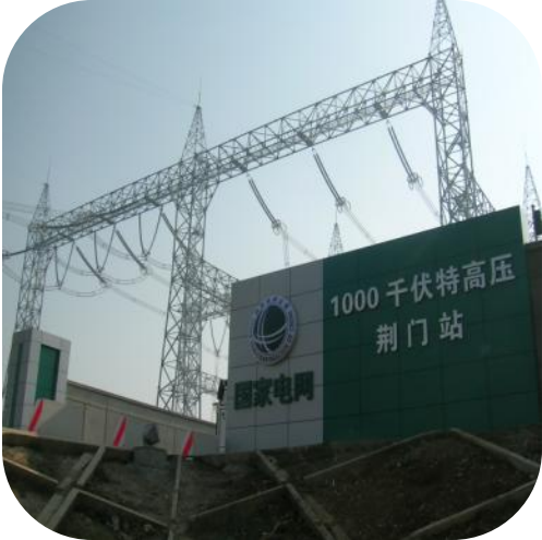
1000kV HVAC Transmission Protection & Automation
