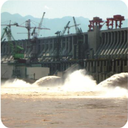
Three-George Hydro Generation Protection & Control
