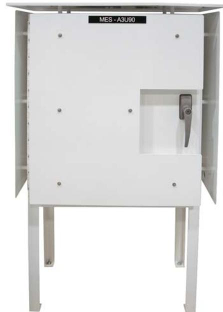
Fig. 13. New outdoor I/O module cabinet
