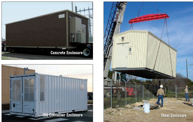
Fig. 12. Substation control enclosures
