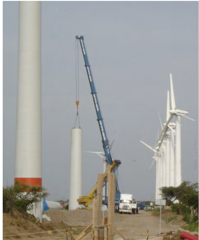
Fig. 16. Construction of the wind farm
