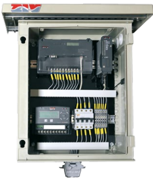
Smartgrids cabinet Compact CCT with WAN communication (pole mounted distribution transformer)
