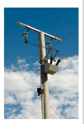
Outdoor smart control cabinets enable both local actuation over OCR elements and remote control from the system control center via wireless connectivity and control protocols. Battery management and operation support is also available.
